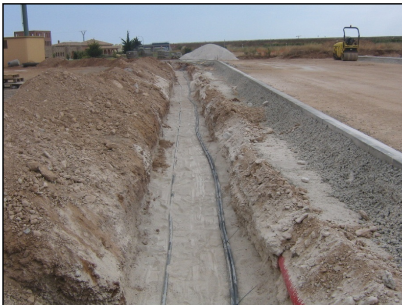
Figure 8: Low-voltage underground cabling
