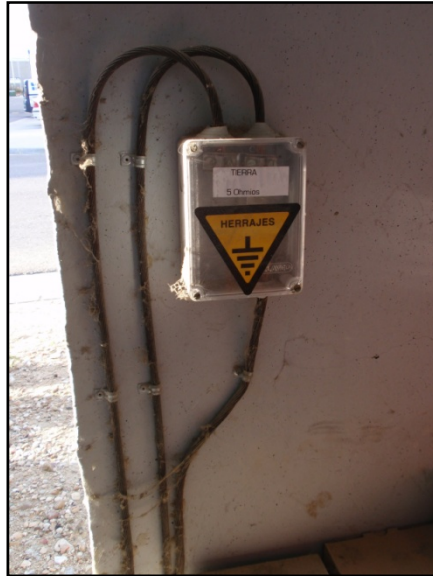
Figure 6: Box for checking the protection ground in the transformer station
