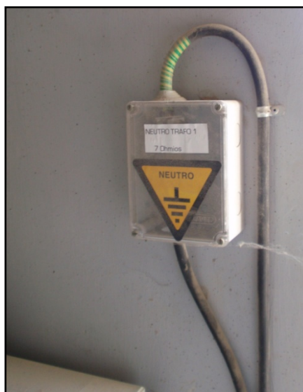
Figure 7: Box for checking if neutral is connected to earth in the transformer
