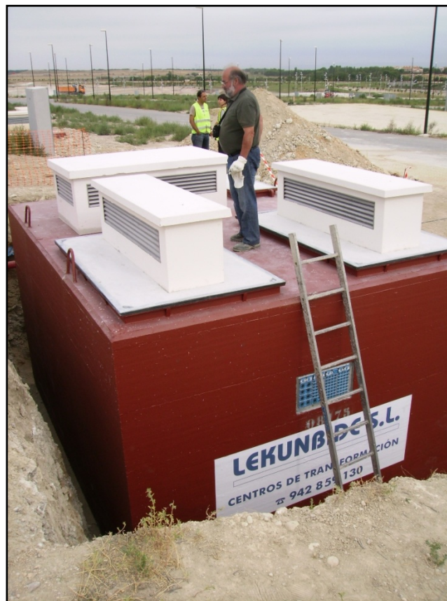
Figure 2: Underground transformer station
