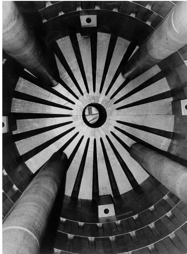
Figure C.7: Top view from of the empty AVR core reactor
