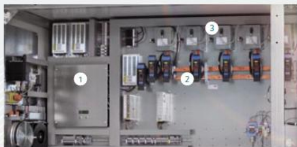
1 Flow-battery-controller (FBC) 2 DC conductor rail 3 Transition from transformer (stacks) to DC
