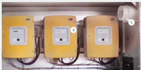
4 Inverter with AC connection 5 Cooling system (ventilation)
