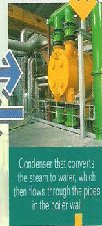
Water is taken from the channel to cool the steam. The water is returned after use
