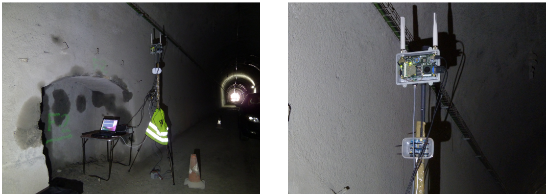
Figure A.4: Mapping wireless coverage - Somport Tunnel
