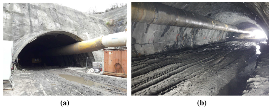
Figure A.13: Tunnel under construction Durango-Amorebieta.
