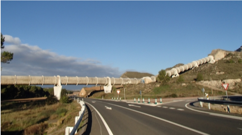
(a) Straight and tilted parts of the pipe
