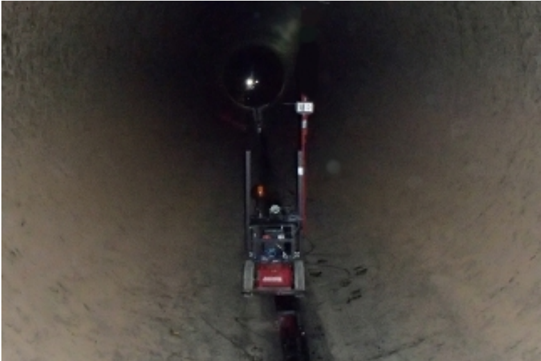
(b) Instrumented Pioneer P3AT robot inside the pipe
