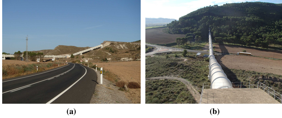
Figure A.6: Santa Ana dam pipe.
