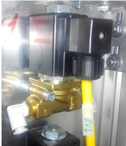
Figure 8.12: Solenoid valve during installation.
