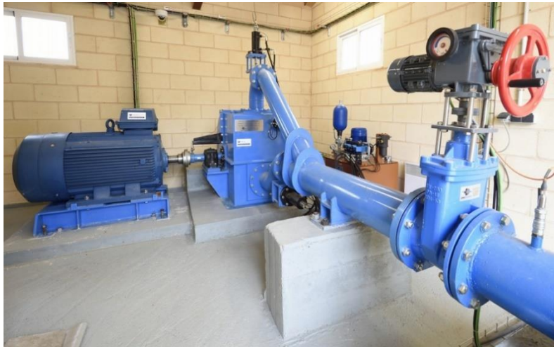
Figura 29, turbina Pelton
