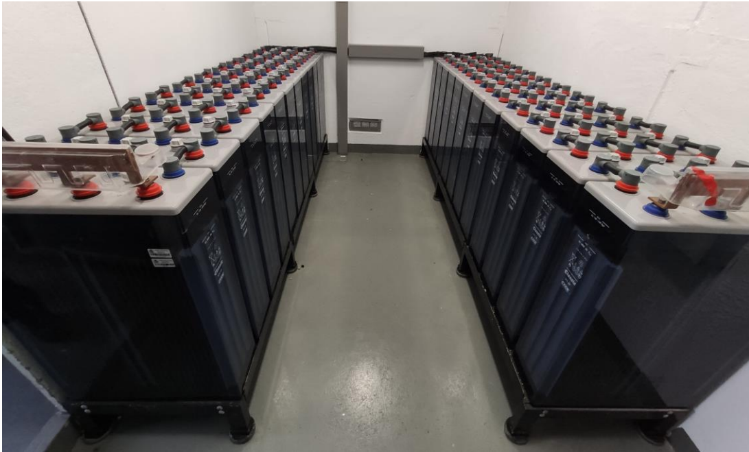
Fig. 1.3. VRLA-based ESS in a photovoltaic standalone installation
