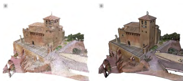
Figure 11. WebGL environment: point cloud visualization of the Santa Tecla church (Cervera de la Cañada, Spain) with different rendering features.
