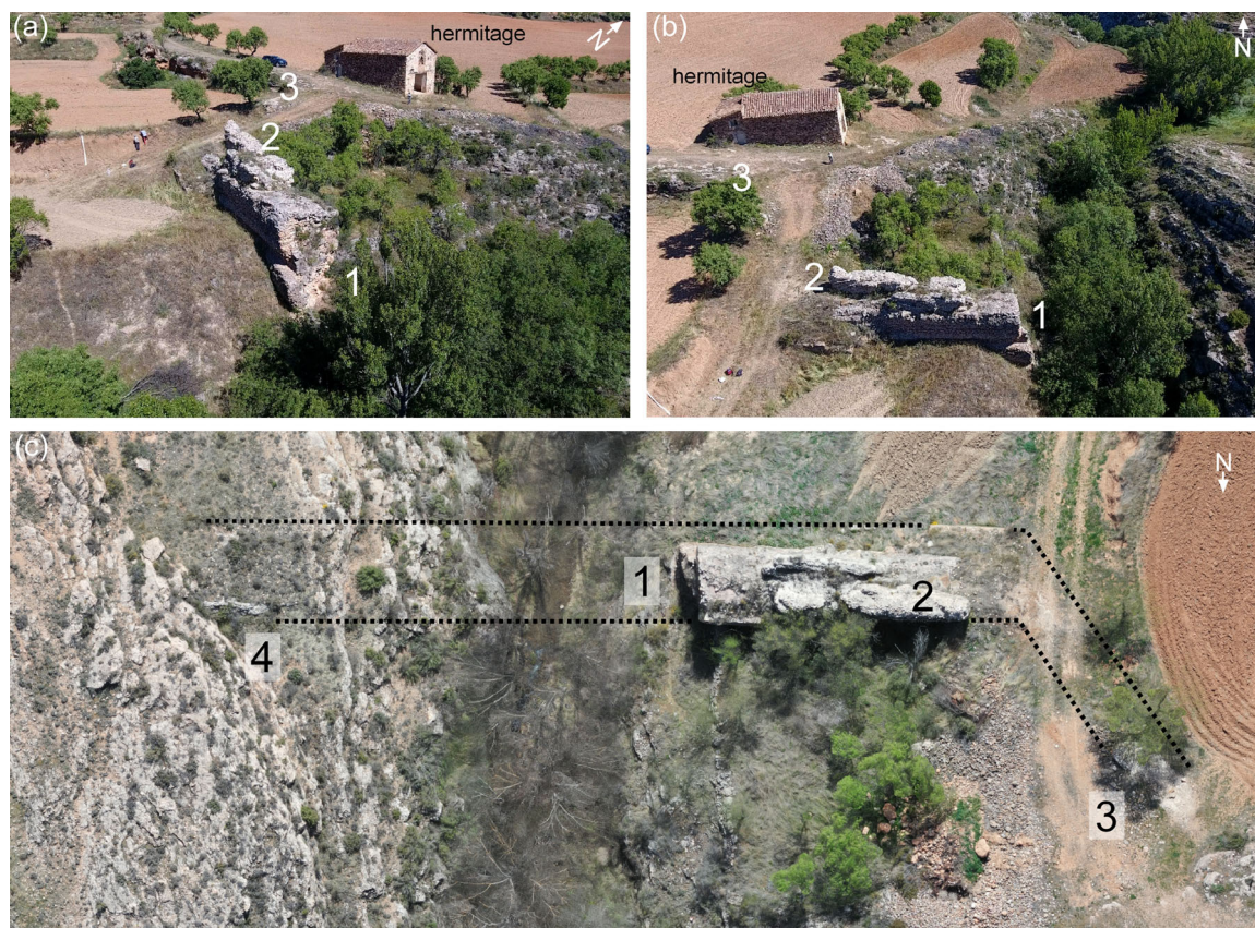
FIGURE 4 Remains of the Monforte dam from (a) side; (b) front; and (c) overhead perspectives. Numbers represent the observed sectors: (1) original dam; (2) extended wall; (3) lateral extension and redirection and (4) remains from the right riverside.
