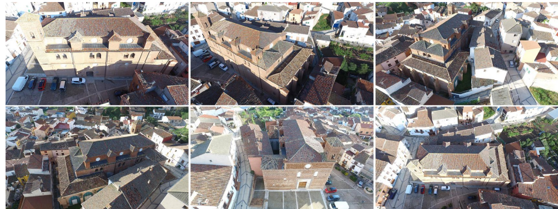
Fig. 7 - Photogrammetric survey carried out with UAV in a difficult accessibility environment. Church of Santa María (Tobed).
