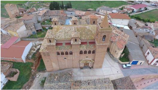
Fig. 3 - Photograph taken with an unmanned aerial vehicle (UAV) of the exterior of the Church of San Félix (Torralba de Ribota).
