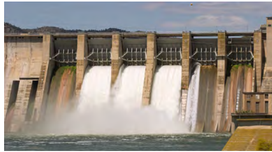
Figure 6. Front view of the Mequinenza dam. [Source: CHE].
