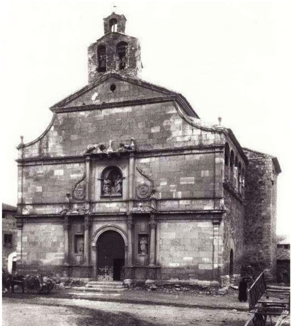
Fig. 5 Frontal façade of the Used parish church in 1947, showing the bell tower that collapsed during the earthquake of 1953 (source: Archivo Mas)
