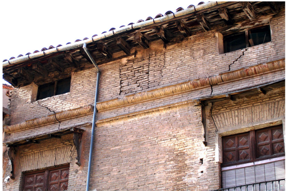
Fig. 6 Symmetrical cracks in the façade of a building in Calle Mayor of Daroca town
