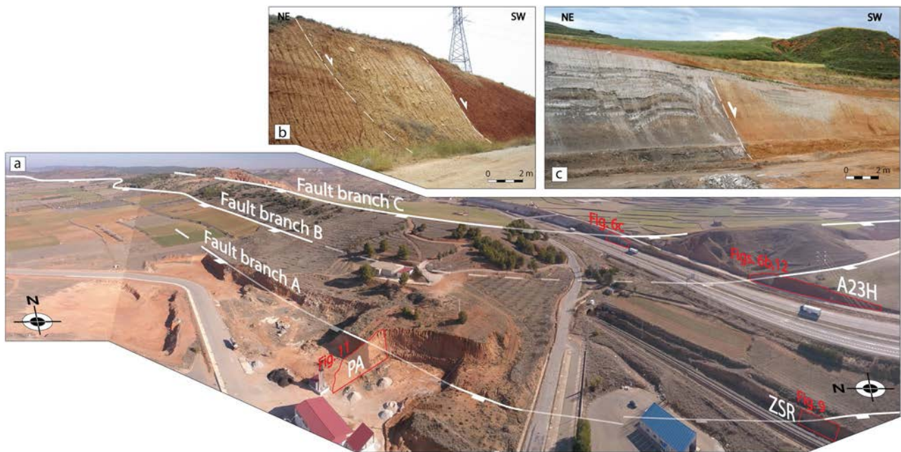
Fig. 6 a Oblique aerial view of the area east of Calamocha town, where the traces of fault branches A, B and C representing the central sector of the Calamocha fault zone are drawn. b Branch B exposed
