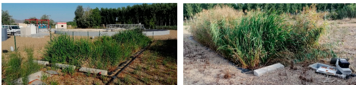
Figure 7. Images of constructed wetlands in summertime. On the (left), FWS pond with reed and bur reed (the installation for air pumping is observed along the right side). On the (right), HSSF pond with reed, with the sample collection device in the foreground.
