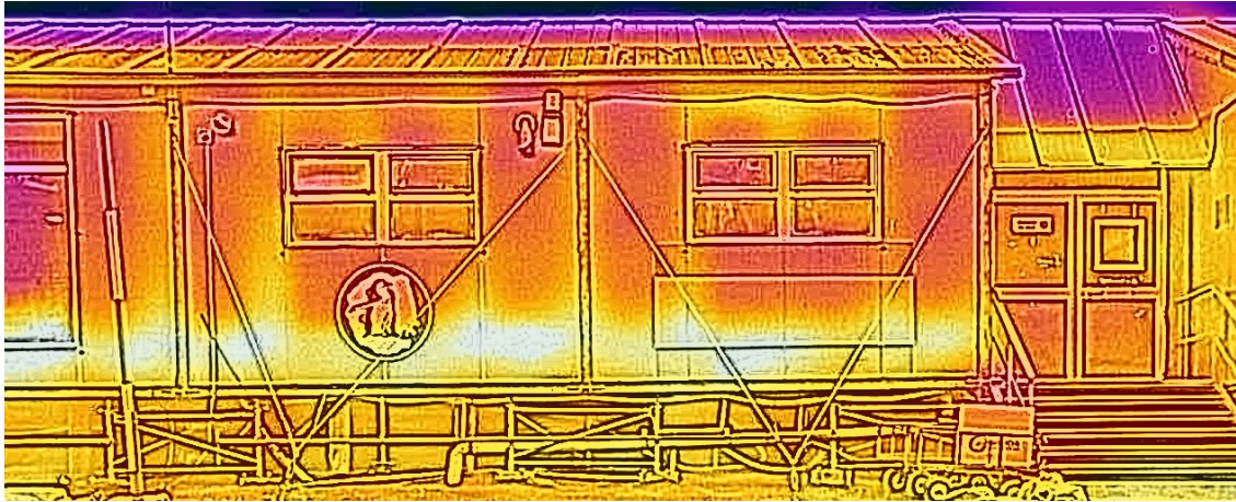
Figure 15. Exterior thermography of the living wing: deterioration of frontal wall insulation.
