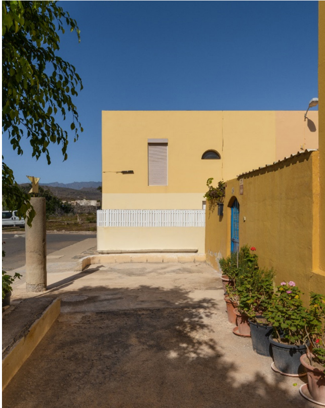
Image 1. 30 social houses in Juan Grande, Gran Canaria. Design by Magüi González (1983-1986). Current state of the small square in the recess of the central rows: on the left, one end of the continuous bench and one of the pedestals with a sculpture by Peleteiro can be seen. Source © María Rodríguez Cadenas (2023).
