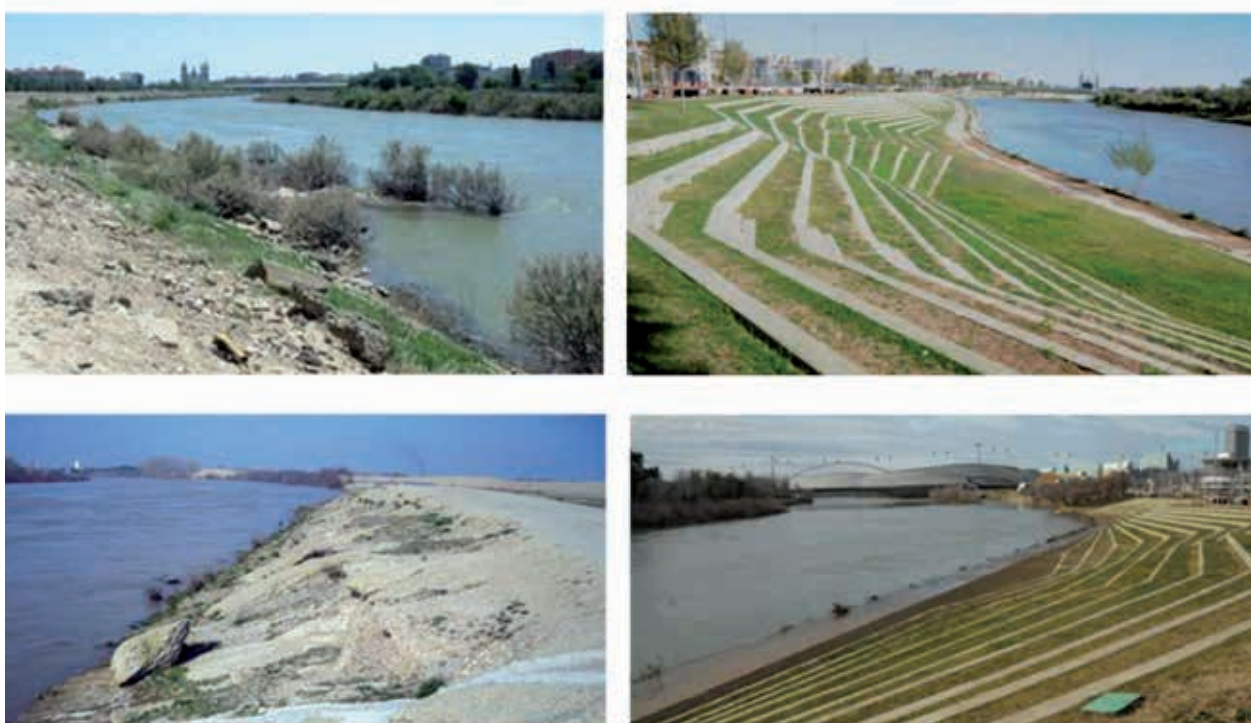
Fig 34. Expo riverfronts before and after the International Exhibition. Source: Pablo de la Cal
