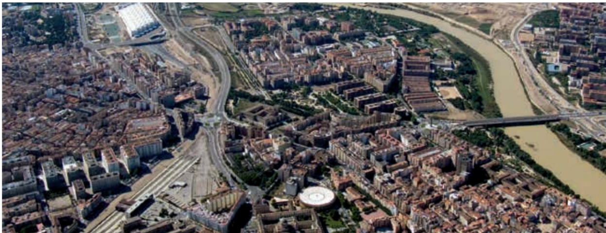
Fig 16. Aerial view of the rail land area and the Expo site in progress, 2006. Source: ZAV.
