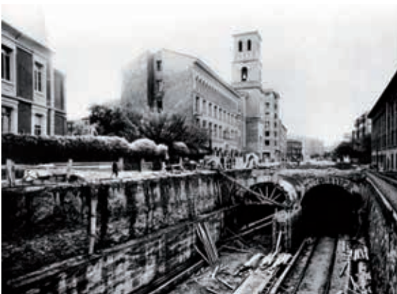
Fig 5. The process of tunneling the railway across the city, 1970s. Source: Flickr.com
