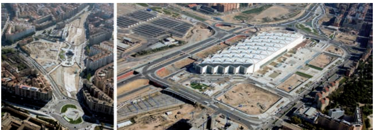
Fig 29. Works at Portillo and Delicias areas in 2008, during the Exhibition. Source: ZAV.
