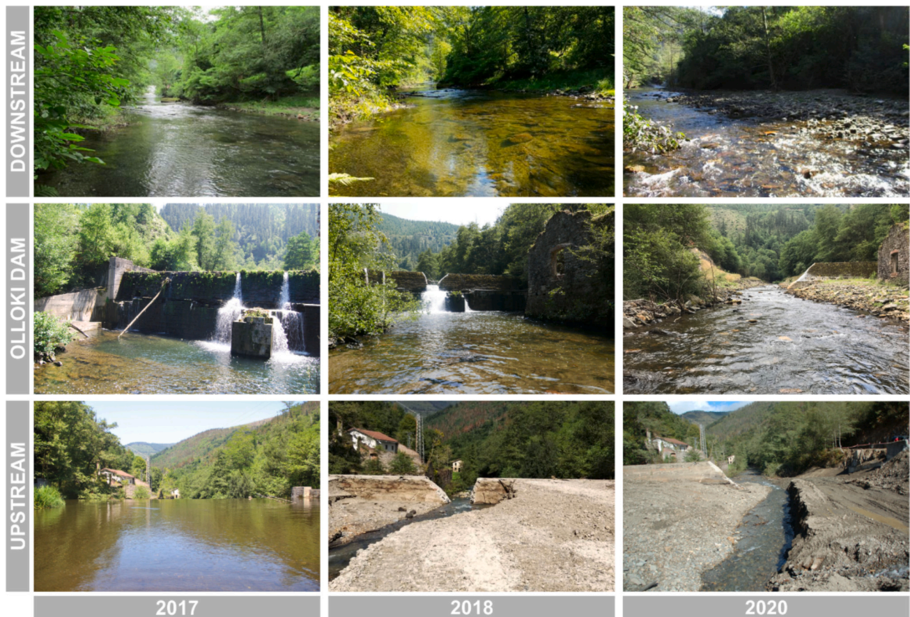
Fig. 2. Images showing the Olloki dam (photos taken from downstream to upstream) and the river immediately upstream (photos taken from upstream to downstream) and downstream the dam, before the removal (July 2017), partial removed (September 2018) and completely removed (July 2020) (photos taken from downstream to upstream).
