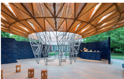
Figura 2.2.4: Pabellón Serpentine Gallery 2017, Londres.
