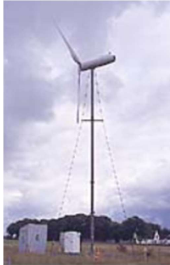
Fig. 20. Guyed wind tower (Danish wind industry association)
