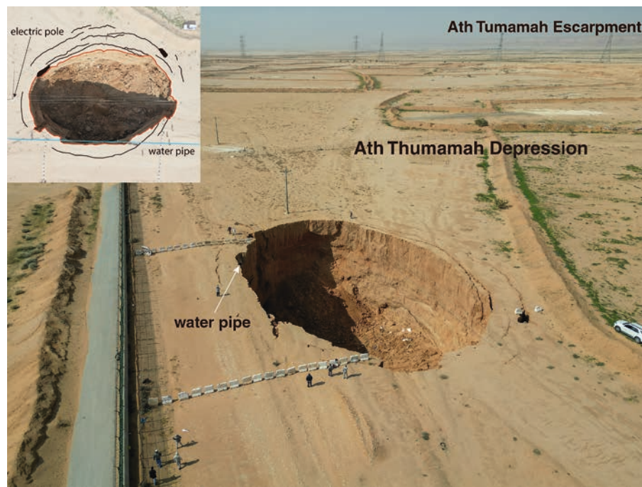
Fig. 13. Expanding cover and bedrock collapse sinkhole 50 m long in the Ath Tumamah depression occurred between December 2017 and July 2019 and associated with a water pipe. The sinkhole is located at the SE projection of the Ath Thumamah fold scarp, suggesting its association with a buried dissolution front (38R 679611E 2,782,485 N).
