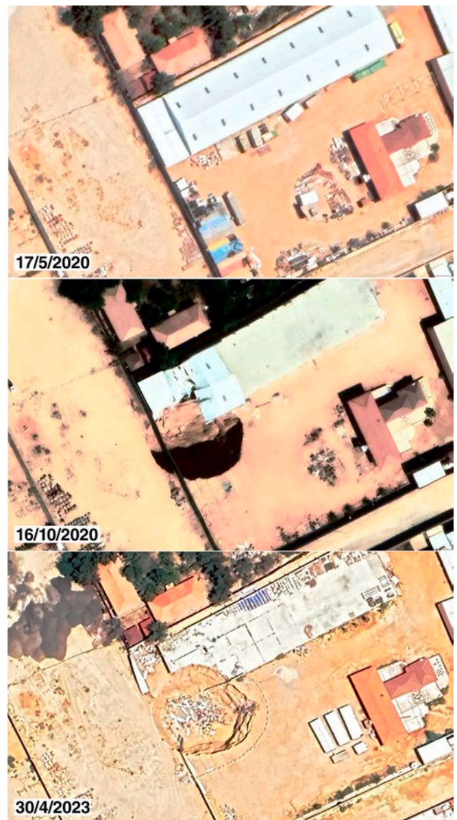
Fig. 26. Collapse sinkhole that occurred in May–October 2020 around 2.7 km southeast of Dahl Hit, resulting in the destruction of a building (38R 703342E 2,706,868 N). New sinkholes can be expected in this areas subject to massive water infiltration from artificial lakes. Images captured from Google Earth.
