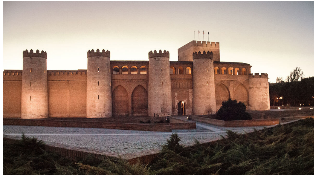
Figure 1. The palace of La Aljafería. Source: adapted from “The Aragonese ephemeris of the day recalls that today, 1 March 1836, ‘El Trovador’ gave his name to a tower of the Aljafería” [39].
