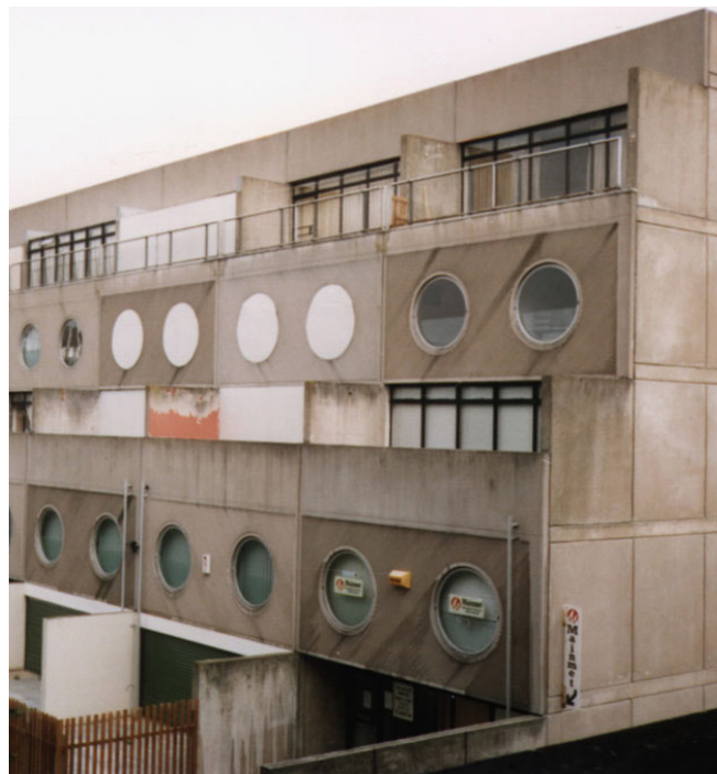
Fig. 43. Southgate Estate , Runcorn, James Stirling, 1977. Fachada bloque tipo, 1985
