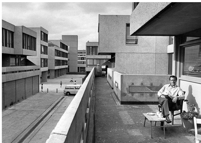
Fig. 37. South Thamesmead, Londres, Robert Rigg, 1967. Calle elevada de los spines blocks, 1970
