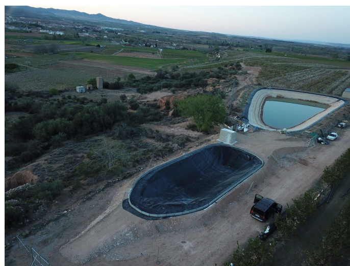
Figure 6. Photograph of the raft just after its construction was completed and before its first filling.
