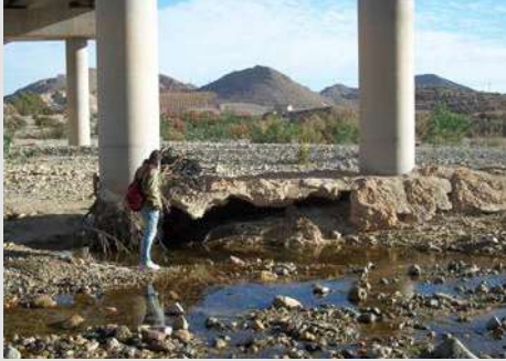
Figures 14 and 15. Bed scouring and removal of the footings of piers supporting the bridge on the AP-7 motorway in the Rambla de las Moreras (Mazarrón, Murcia).
