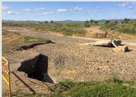
Figures 8 and 9. Culvert pipe of the ford at la Virgen de Lagunas in the Rambla de Cariñena, pulled away by the flood in March 2018. It was the only pipe for the ford in spite of the dimensions of the channel. The ford was destroyed as observed on the right.
