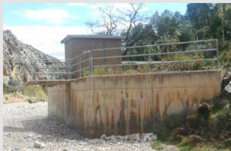
Figure 47. Mouth reach of the Barranc de la Rompuda under the urban district of Orpesa (Castelló). Figure 48. Gauging station of the River Seco (Oliete, Teruel) partially invading the natural channel.
