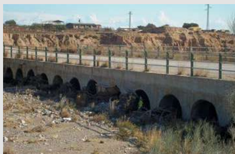
Figures 12 and 13. Left (fig. 12): Bridge-ford provided with culverts and a concrete ramp downstream in the Rambla de La Murta (Murcia). On the right (fig. 13) a close-up of a bridge-ford in the upstream section.
