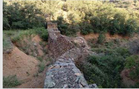
Figure 36. Sedimen retention by a check dam in the Barranco de La Recueja (Alcalá de Júcar, Albacete). Figure 37. Semi destroyed gabion check dam in the Rambla de la Pimienta (Manchones, Zaragoza).
