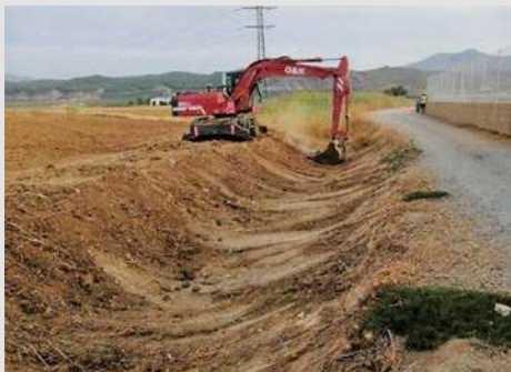
Figure 41. Opening of a drainage cross-section to protect a road in Antequera (Málaga). Figure 42. On the right, results of dredging in the River Cidacos (Arnedo, La Rioja). On many occasions, like in this case, the gravel is not extracted, but rather it accumulates on the channel sides, with the lateral deposits becoming larger and producing the destruction of bed forms and banks.
