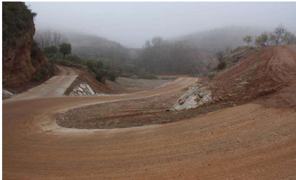
Figure 104. Tracks that have a barrier effect and invade the channel in the Barranco de la Mata (Jubera, La Rioja)
