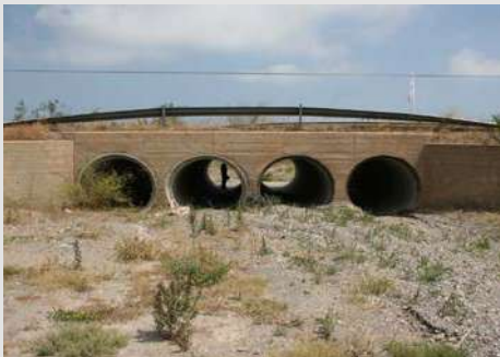
Figure 18. At the intersection of the Rambla de los Pinares and the D14 road (Águilas, Murcia) the culverts present a drainage capacity much lower than is necessary and are often useless because of obstruction. Figure 19. Rambla de la Anchura (Murcia) with local bed scour at the foot of the cement floor.
