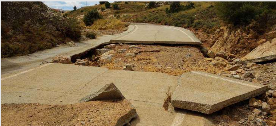
Figures 29 and 30. Two photos of the road joining Corbatón and Alpeñés (Teruel) invading and traveling along the Rambla de Corbatón for one kilometer. In the two images below (figures 31 and 32) we can observe the consequences of flood in August 2020, which destroyed this road.
