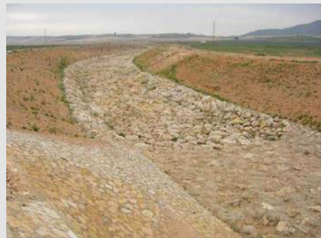
Figures 66 and 67. Two photos of channelling and masonry lining of the bed in the Rambla Mullidar (Liétor, Albacete).
