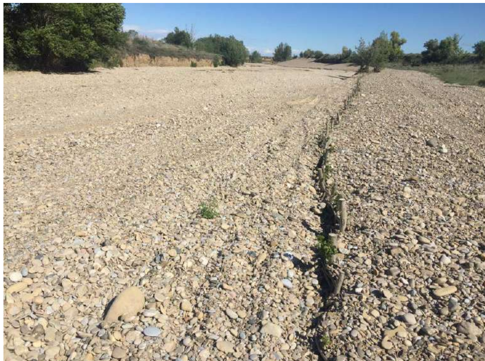
Figure 119. Bad practice of revegetation in a dry channel reach of the Arba de Luesia (Rivas, Zaragoza) altered by recovery work of the drainage cross-section. The aligned stakes narrow the channel.
