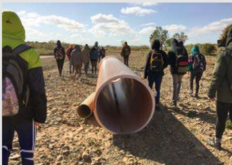
Figures 8 and 9. Culvert pipe of the ford at la Virgen de Lagunas in the Rambla de Cariñena, pulled away by the flood in March 2018. It was the only pipe for the ford in spite of the dimensions of the channel. The ford was destroyed as observed on the right.
