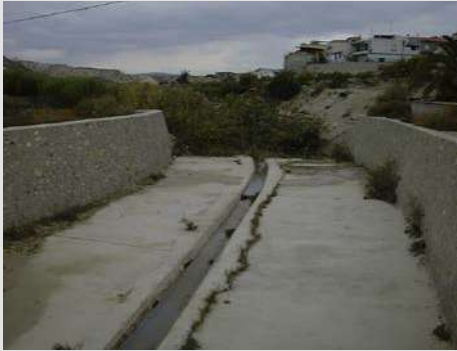
Figures 70 and 71. Reach in Rambla de Albudeite canalised with masonry walls and concrete lined bed (Murcia) and section of the River Campanillas (Málaga) channelled by longitudinal dikes of loose stone.
