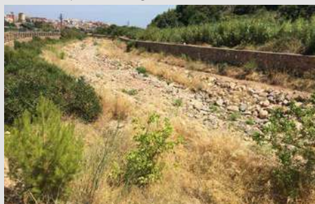
Figures 62 and 63. Channelling with riprap and gabions in the Rambla de Alcofea (Zaragoza) and with walls in the Rambla de Sant Josep in La Vall d'Uixó (Castelló).
