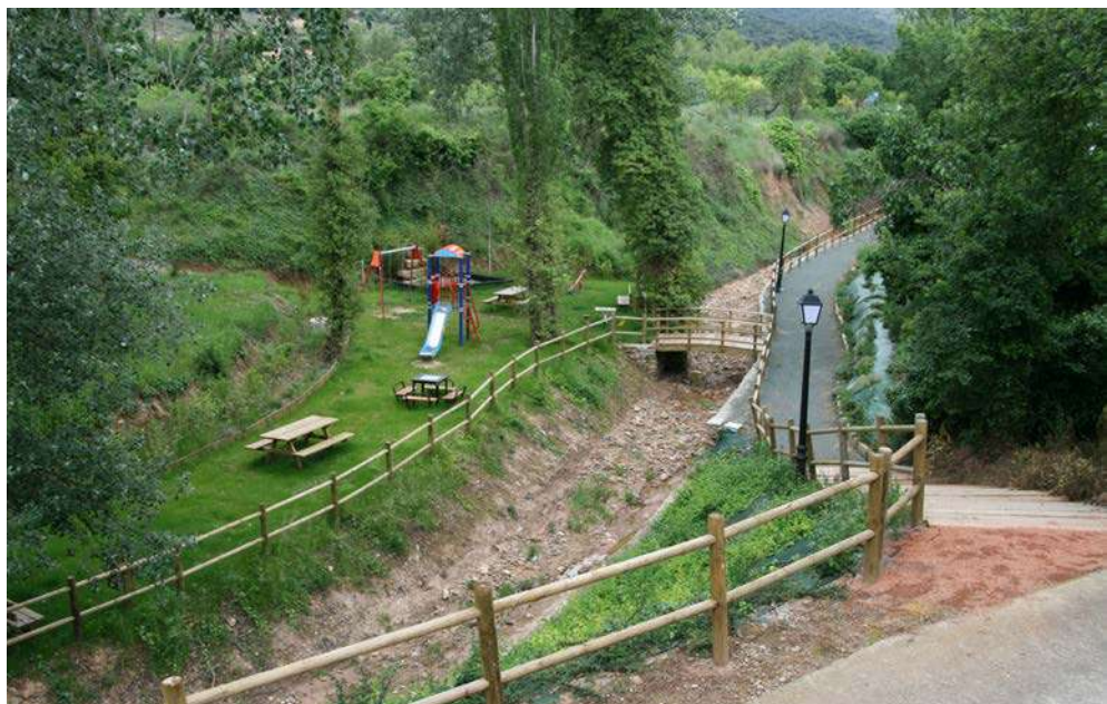
Figure 113. Action of urbanisation and “fluvial park” in the Barranco Valvadera (Bergasa, La Rioja), which has altered its original morphology. We must try to avoid these actions and restore natural geomorphic units.
