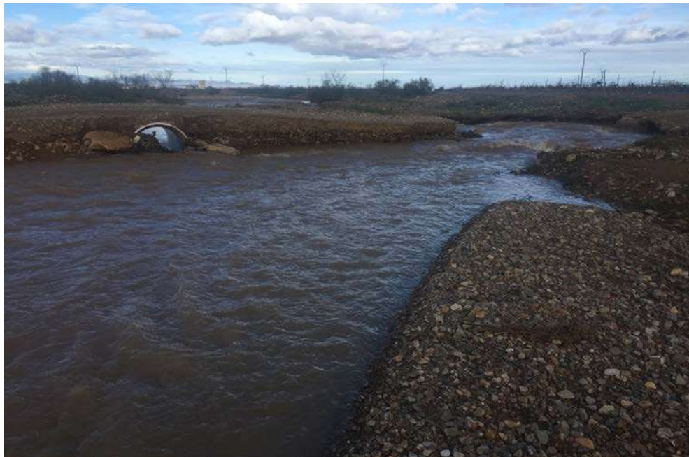
Figure 110. The flood in the Rambla de Cariñena, as a result of the storm Gloria episode (January 2020), destroyed the ford of the Virgen de Lagunas, rendering the only existing pipe under it useless. Apparently, this ford is illegal and it is the local owners who rebuild it after each flood.
