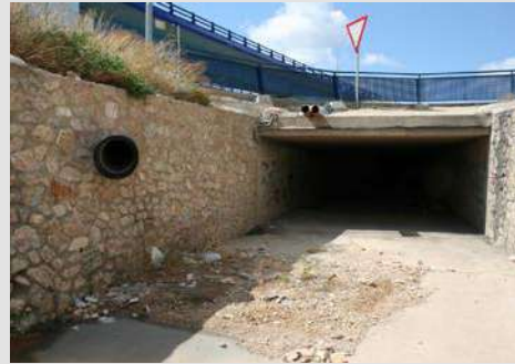
Figure 16. A ford without inferior drainage in the Rambla de la Torre (Perín, Cartagena). Figure 17. Road crossing over the channel connecting the ramblas de los Dolores and Benipila (Cartagena) saved by a reinforced concrete pontoon structure.
