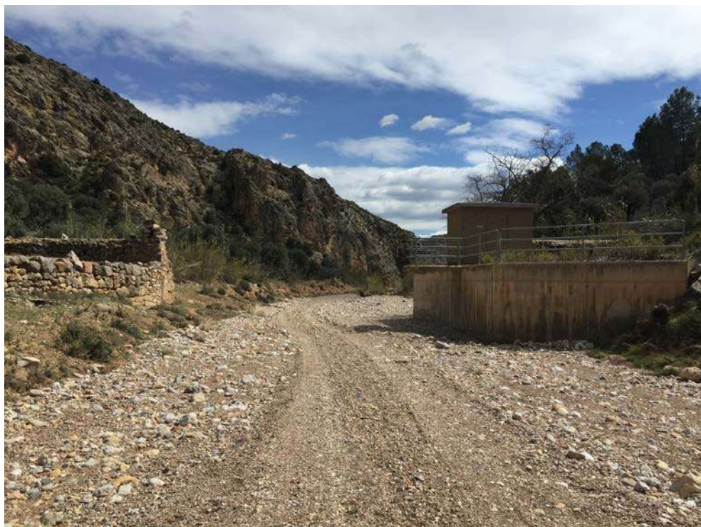
Figure 126. One of the very few gauging stations in the ephemeral network of the Ebro basin, that of the Seco River in Oliete (Teruel), built after the flash flood of 2013, which caused a fatality.
