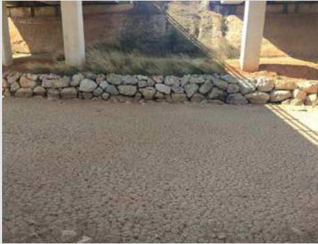
Figure 64. Stone riprap protecting the bridge pillars at the highway crossing on the Rambla de las Balsas (Longares, Zaragoza). Figure 65. Removal of defences in an incised channel reach in the Rambla de las Moreras (Mazarrón, Murcia).
