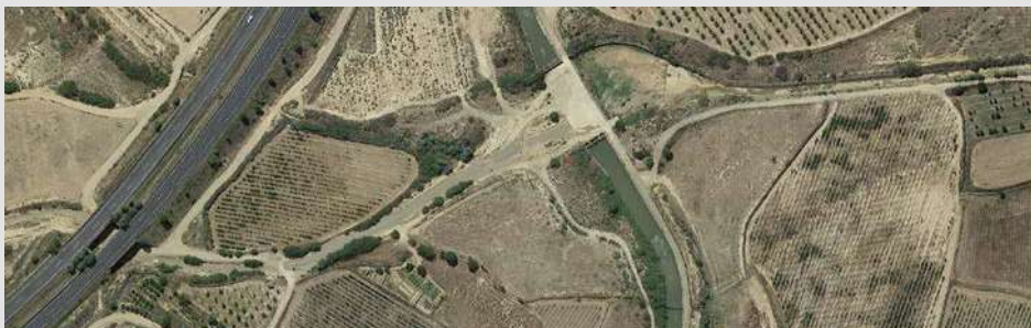
Figure 80. Lower reach of la Yasa Agustina stream (Aldeanueva de Ebro, La Rioja) with a rectification to the channel so that it can pass over the Lodosa Canal.
