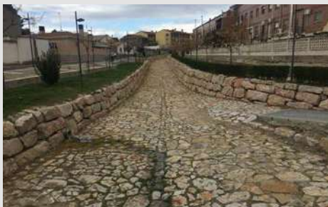
Figure 60. Canalisation of the Barranco de las Casas in la Puebla de Alfindén (Zaragoza) whose reform in 2014 reduced the channel flow capacity by at least half. Figure 61. Canalisation of the Riera de l'Alforja (Tarragona).
