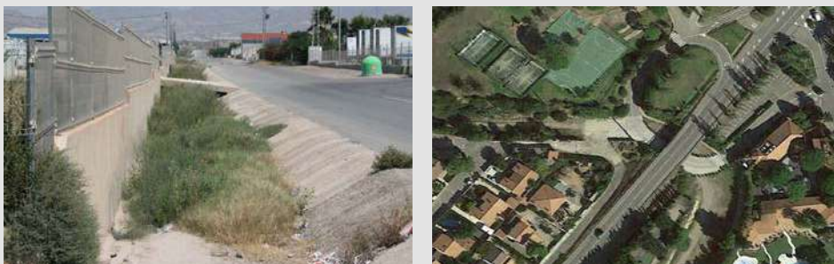
Figure 27. The N-332 road occupies the Rambla del Charco (Cartagena) and has been raised leaving the channel as a small ditch. Figure 28. The Barranco de la Porquerola is partially occupied by an access road in the housing estate in Montroig del Camp (Tarragona).
