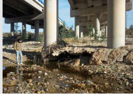
Figures 14 and 15. Bed scouring and removal of the footings of piers supporting the bridge on the AP-7 motorway in the Rambla de las Moreras (Mazarrón, Murcia).
