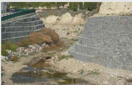
Figures 62 and 63. Channelling with riprap and gabions in the Rambla de Alcofea (Zaragoza) and with walls in the Rambla de Sant Josep in La Vall d'Uixó (Castelló).
