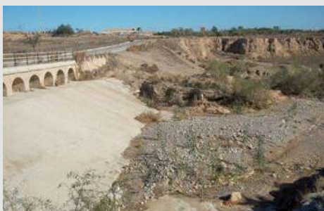
Figures 12 and 13. Left (fig. 12): Bridge-ford provided with culverts and a concrete ramp downstream in the Rambla de La Murta (Murcia). On the right (fig. 13) a close-up of a bridge-ford in the upstream section.
