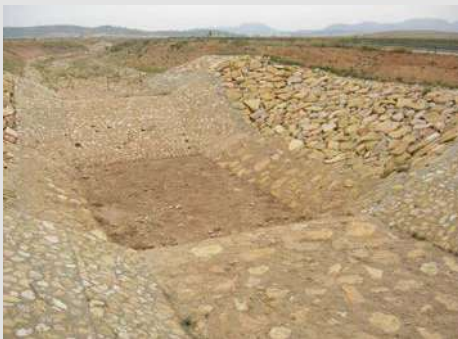
Figures 66 and 67. Two photos of channelling and masonry lining of the bed in the Rambla Mullidar (Liétor, Albacete).
