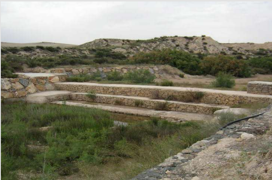
Figure 35. Weir that takes water from the Rambla de Torrealvilla (Lorca, Murcia).
