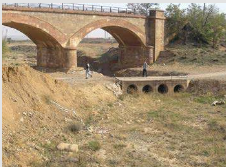
Figure 10. Bridge and road-crossing drainage culverts in the Rambla de Valdemorado in Cariñena (Zaragoza). Figure 11. The crossing of a simple path can modify the local base level and alter the longitudinal profile of an ephemeral stream (Sierra de Armantes, Zaragoza).
