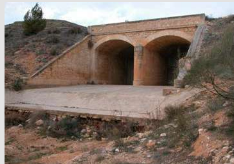
Figure 18. At the intersection of the Rambla de los Pinares and the D14 road (Águilas, Murcia) the culverts present a drainage capacity much lower than is necessary and are often useless because of obstruction. Figure 19. Rambla de la Anchura (Murcia) with local bed scour at the foot of the cement floor.
