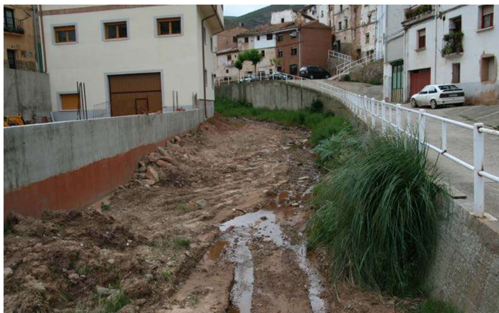
Figure 124. Barranco Valera in Herce (La Rioja)
