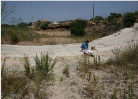
Figure 16. A ford without inferior drainage in the Rambla de la Torre (Perín, Cartagena). Figure 17. Road crossing over the channel connecting the ramblas de los Dolores and Benipila (Cartagena) saved by a reinforced concrete pontoon structure.
