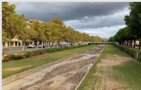
Figure 60. Canalisation of the Barranco de las Casas in la Puebla de Alfindén (Zaragoza) whose reform in 2014 reduced the channel flow capacity by at least half. Figure 61. Canalisation of the Riera de l'Alforja (Tarragona).
