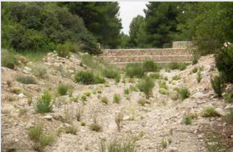
Figure 38. Local scouring and bed armoring downstream of a check dam in the Rambla de Zarzadilla (Murcia). Figure 39. Another example accompanied by the plantation of poplars in the Rambla del Boquerón (Murcia) (right).
