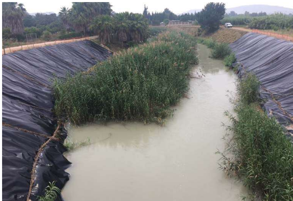
Figure 115. Example in a permanent river (River Segura in Molina de Segura, Murcia) of treatment for the elimination of reeds on both channel banks.
