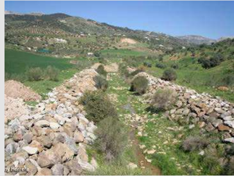
Figures 70 and 71. Reach in Rambla de Albudeite canalised with masonry walls and concrete lined bed (Murcia) and section of the River Campanillas (Málaga) channelled by longitudinal dikes of loose stone.
