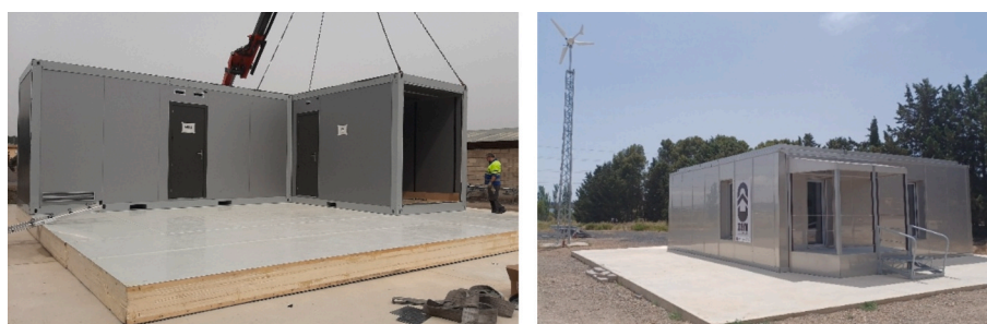
Fig. 2. ZEM prototype during commissioning (left) and demonstration (right) at the Sapper Battalion I, Zaragoza.
