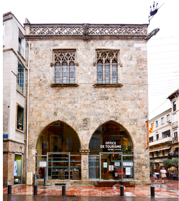
Fig. 3. Guillem Sagrera. East facade, Lonja del Mar, Perpignan (photograph by the authors).
