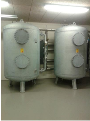
Figure 19: TFB25 filters in Sabro waterworks for cleaning water
