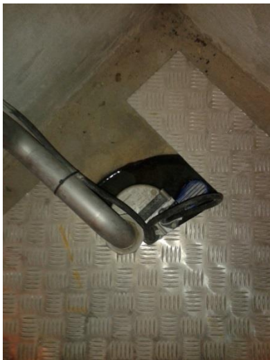
Figure 24: Drainage pump
