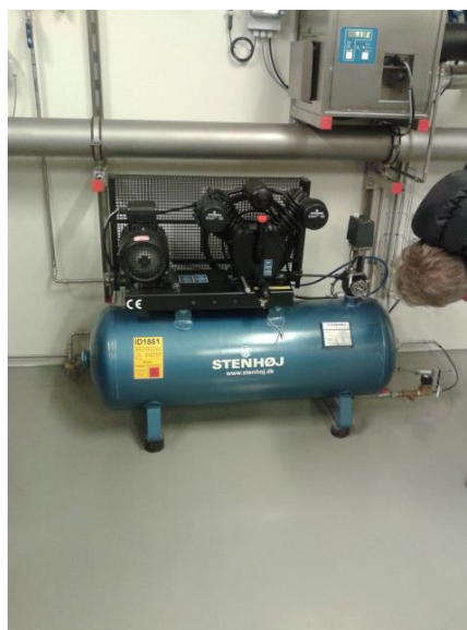
Figure 21: Air compressor for mechanical aeration in filters and for valves
