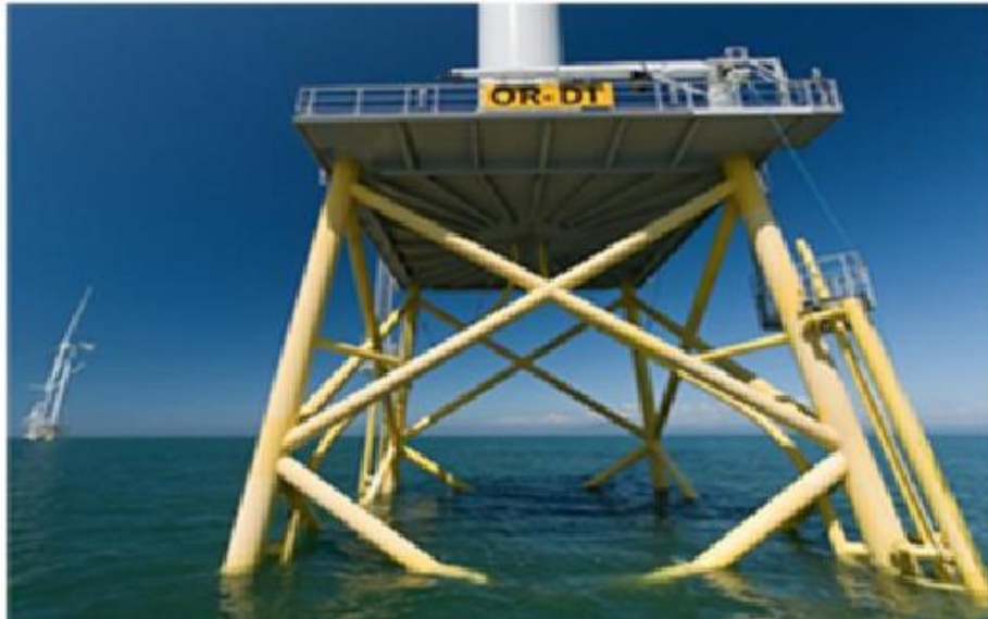
Figure 21: Jack foundation (OWEC Quattropod®)
