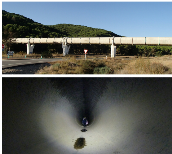
Figure 2.4: Large-scale scenario. Drainpipe (4-m diameter, 300-m length) at the Santa Ana dam (Castillonroy, Spain).
