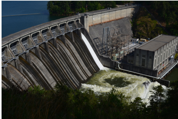
(a) Allatoona dam and lake
