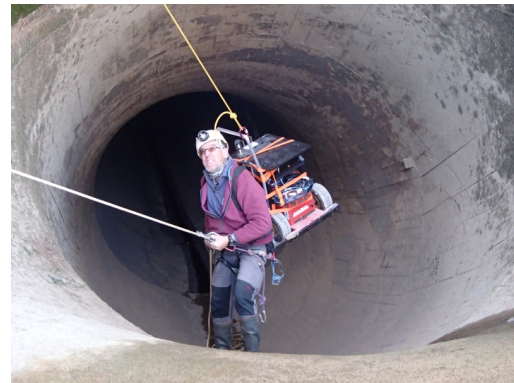
(a) The Santa Ana dam drainpipe from the out- (b) Accessing the pipe with climbing equipment side
