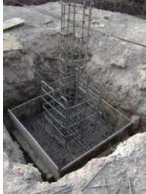
Figure 9. Construction of single footing
