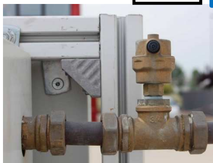
Automatic Vent valve (customer supply)
