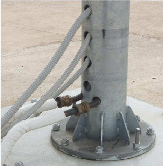
Way out path of cables at the bottom of the pole
