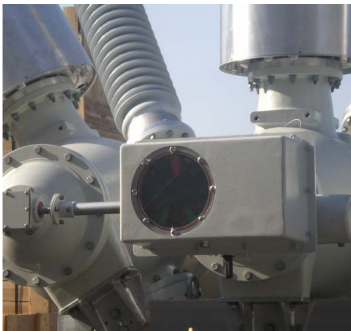
Fig. 6: New disconnector drive mechanism
