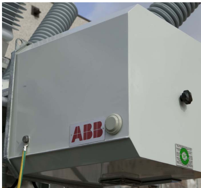
Fig. 5: BLK 222 Circuit-breaker spring drive
