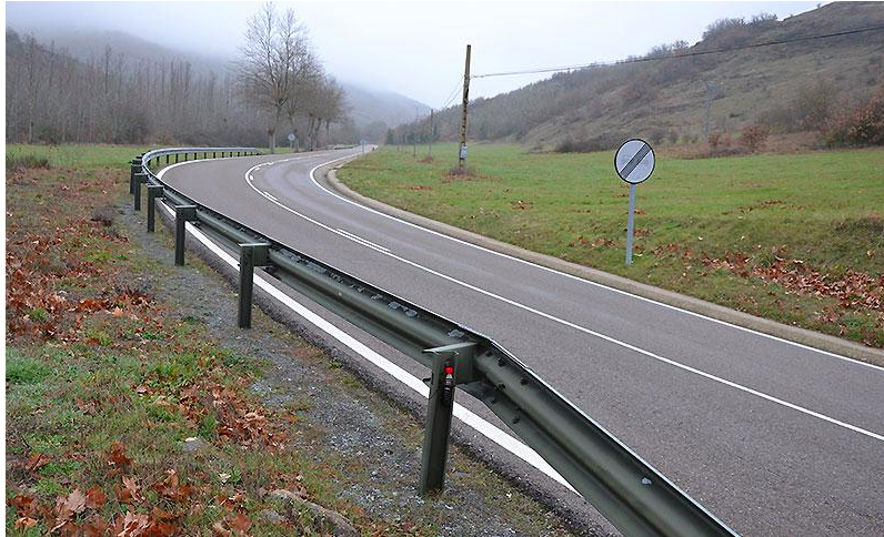
Figure 1. Steel traffic barrier to keep vehicles inside roadway. [2]
