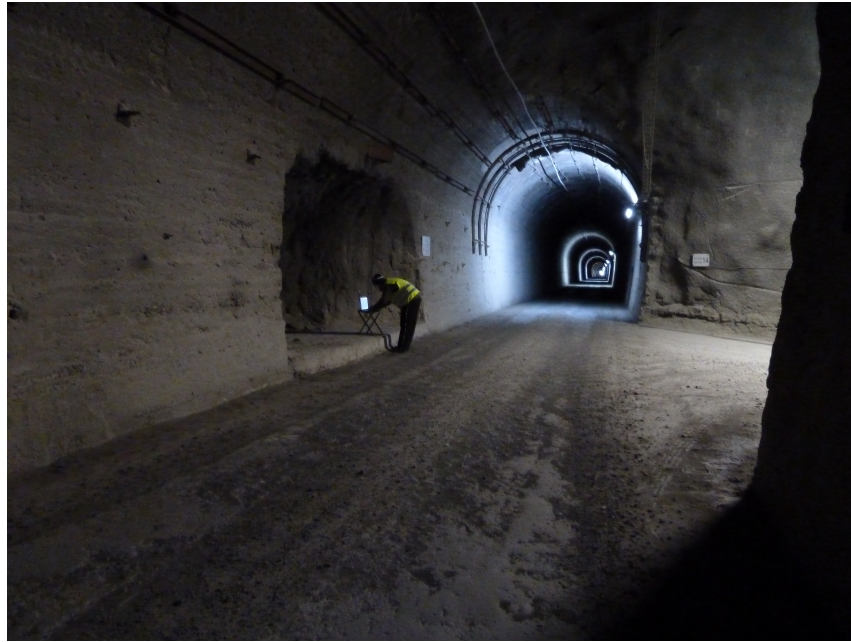
(a) The Somport tunnel at the intersection with Gallery 14 where Router 2 was located
