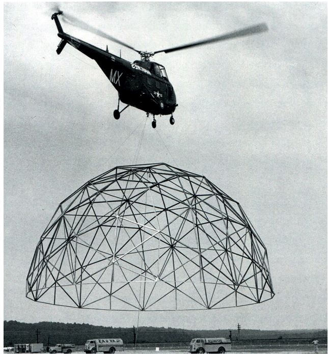
f.6_ Buckminster Fuller U. Marine Corps transporting a dome via helicopter 1954
