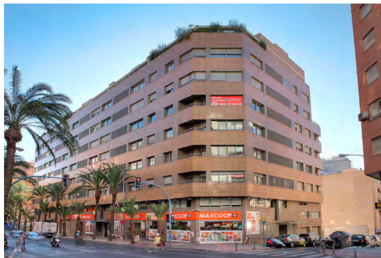
Figure 3. Building façade. North façade and west façade.
