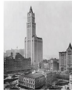
Woolworth Building (Cass Gilbert, 1913), Nueva York. [J]
