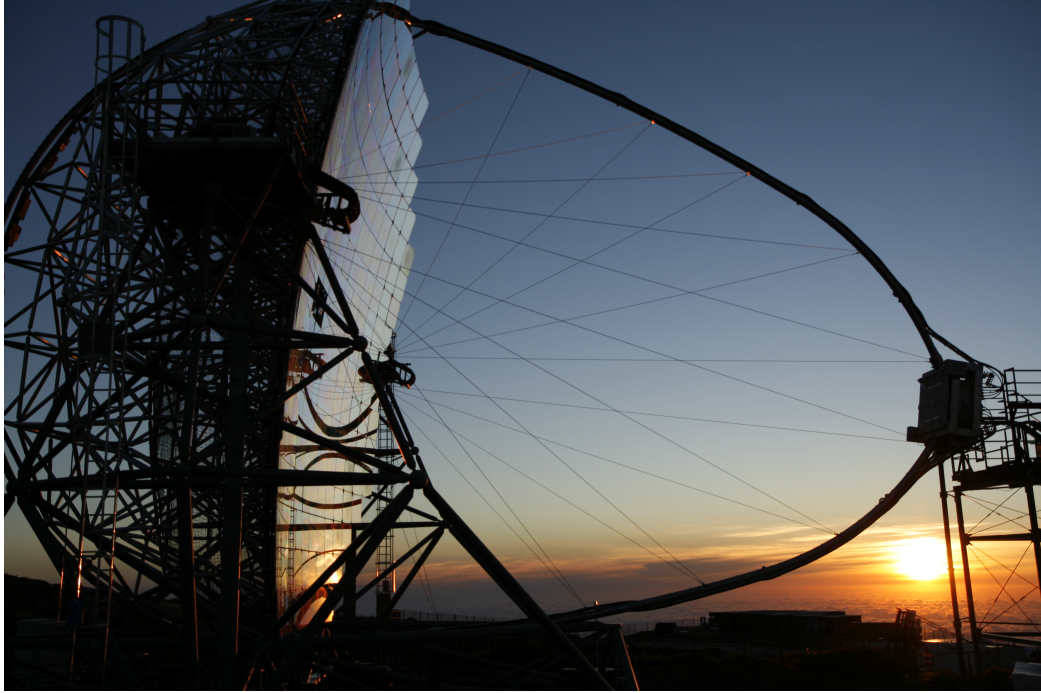
Figure 4.2: Picture of the profile view of the MAGIC II telescope in parking position. On the left, the mirror structure and reflecting surface, on the right, the camera resting on the access tower. Credit: Dr P.Peñil.
