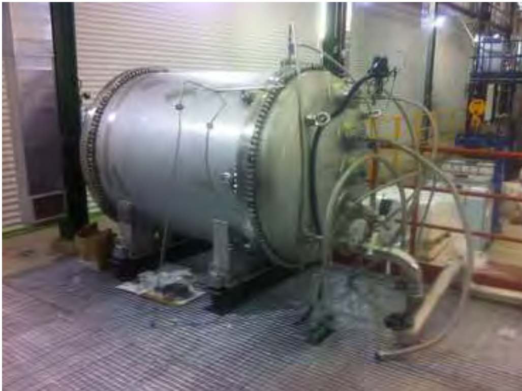
Figure 21: The NEXT-100 pressure vessel is used as expansion tank during the operation of the NEXT-White detector. A new expansion tank with a volume ten times larger will be installed for the operation of the NEXT-100 detector.
