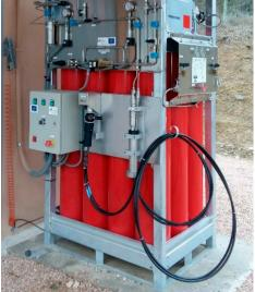
Figure 8. The hydrogen tank and the refuelling system.
