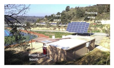
Fig. 3. Assembling of the different solar arrays and main project booth at the WWTP + IS area.
