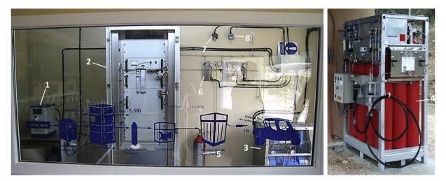
Fig. 5. Hydrogen production and refueling plant. Pictures of the production devices assembled inside the booth and the stationary GSS placed outside (right).
