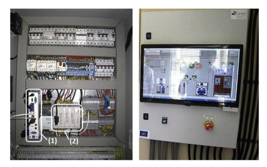
Fig. 4. Inside (left) and outside (right) images of the main control cabinet.
