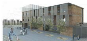
Vista entrada | Entrance view
