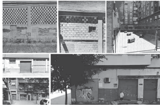
Locales cerrados y espacios sin uso | Closed commercial premises and unused spaces
