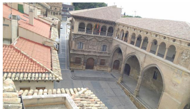
Figure 1. Exterior from the Town Hall of Alcañiz (Teruel)
