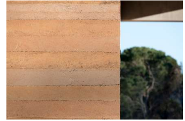
Fig 106 Textura muros de tapial. Fuente: https://www.fosterandpartners.com/projects/narbo-via/#construction
