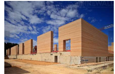
Fig 107 Muros SIREWALL. Fuente: https://sirewall.com/project/narbo-via-history-museum-france/
