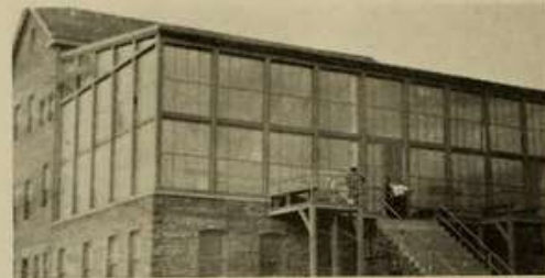
Southern View of the New Solax Building, Showing Studio Proper. All Window Sashes Are Removable.
