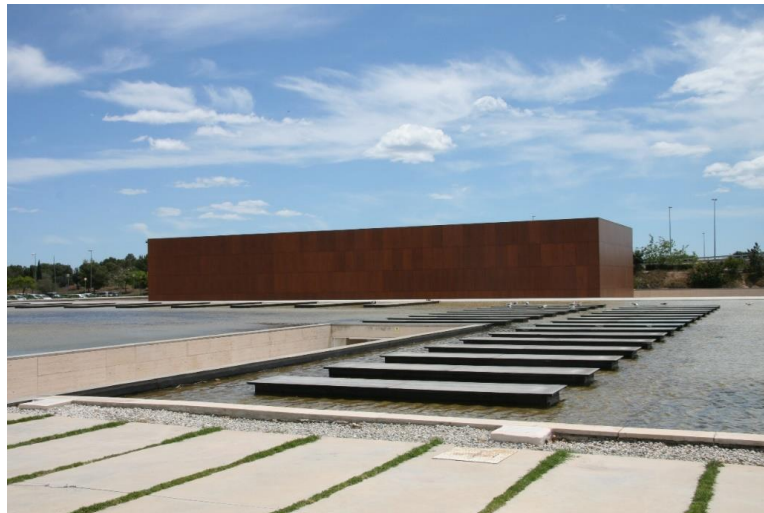
Figure 3. Image of the Museum of the University of Alicante (MUA). The Sempere Hall is below the water-covered roof, on the left.
